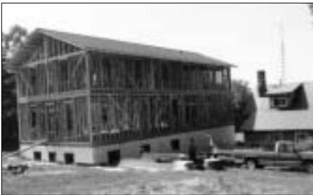
Renovations at Assumption Farm
