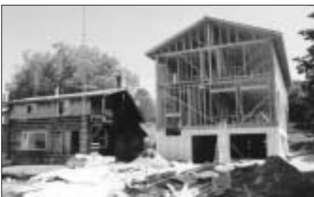
Work in progress at the farm
